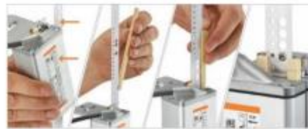
Figure 13: Sensor and Tape Installation
