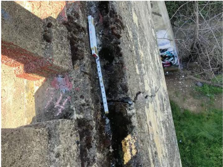
Photo #16 Vertical crack in Girder 4 in Span 1 opening to the top.
