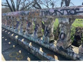
Photo 11 Failed patches in the left bridge rail.
