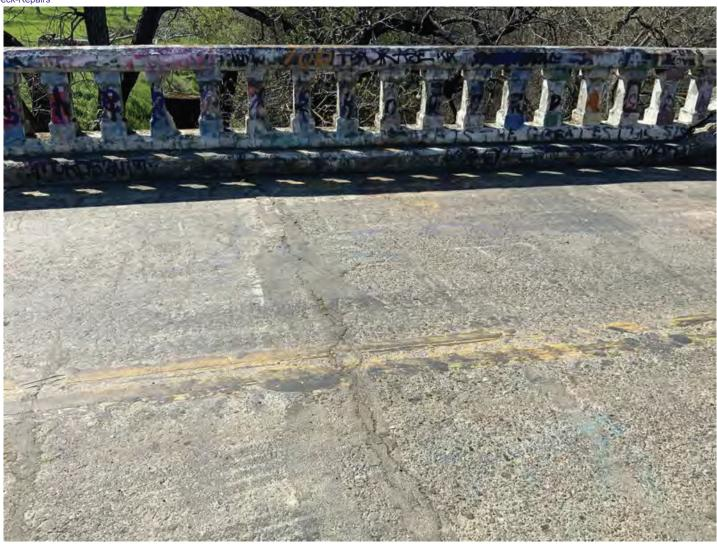
Photo #10 Sealed transverse deck crack in Span 1.
