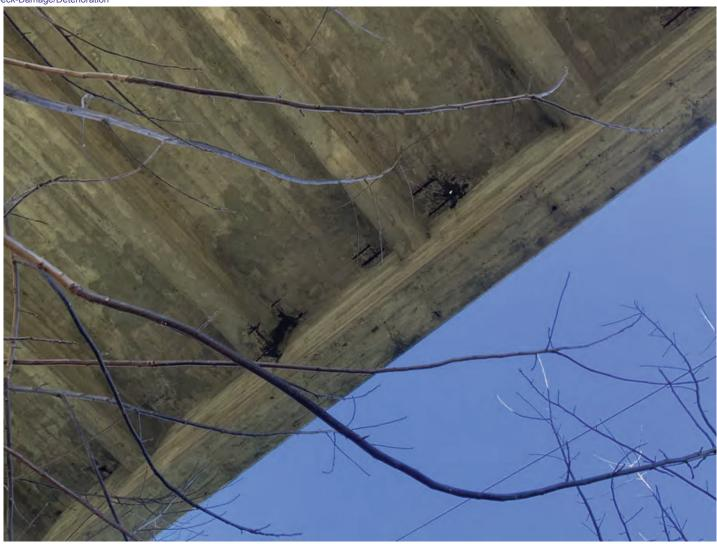
Photo #22 Spalls with exposed rebar in the soffit.
