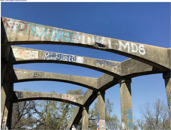
Photo #19 Spall in the first arch strut.
