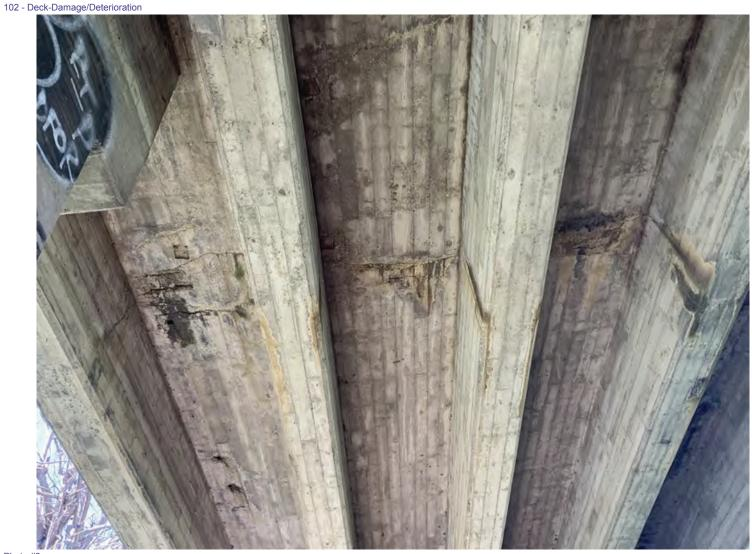
Photo #9 Transverse crack with spalling in the soffit of Span 4.
