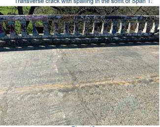
Photo 10 Sealed transverse deck crack in Span 1.
