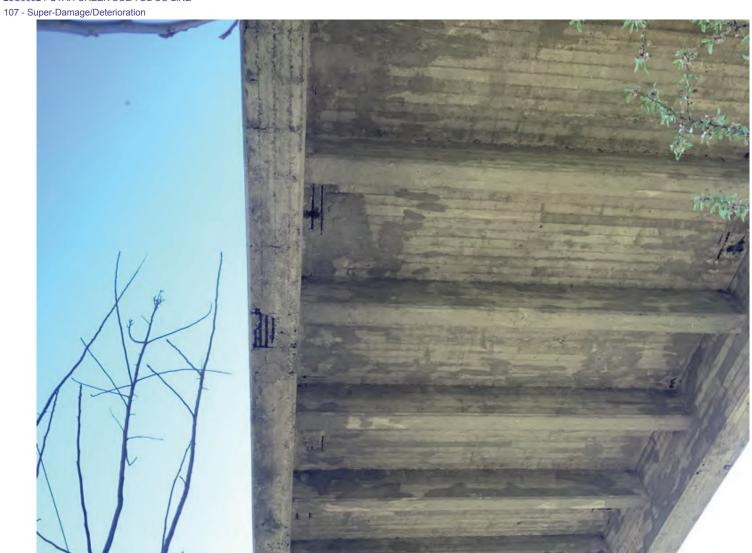
Photo #12 Spalls with exposed rebar in the bottom of the girders.
