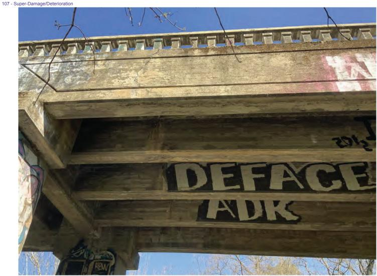
Photo #15 Vertical cracks in the girders in Span 1.
