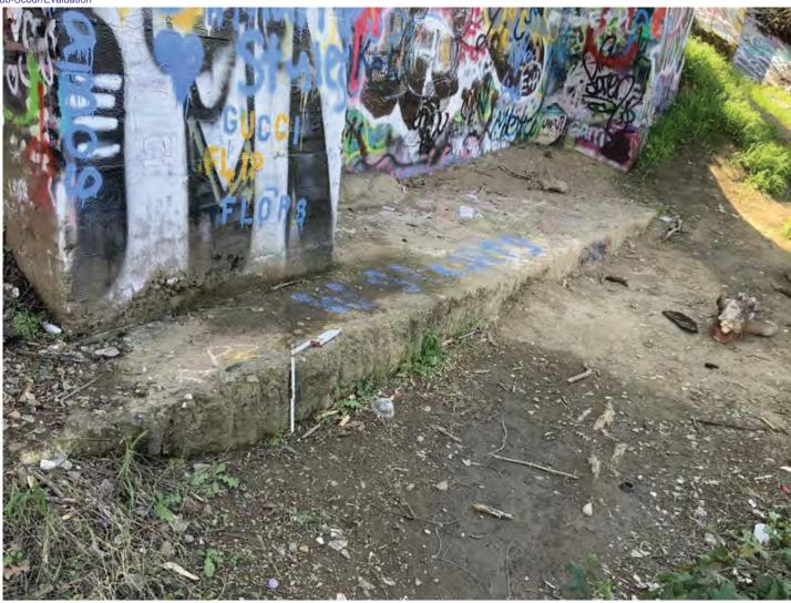
Photo #20 Exposed pile cap at Bent 2.
