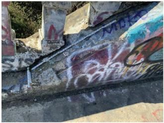
Photo 17 Spall in the left arch rib at Bent 2.
