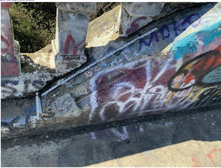
Photo #17 Spall in the left arch rib at Bent 2.
