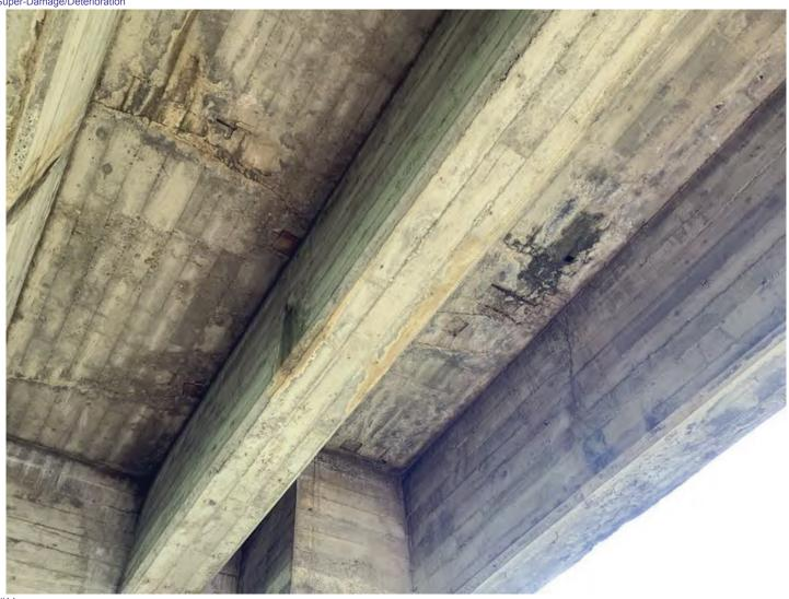
Photo #14 Vertical cracks in the girders in Span 4.
