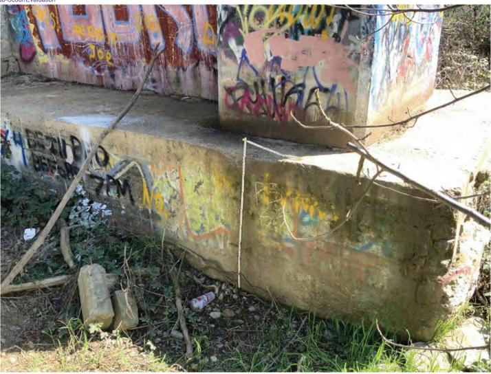
Photo #21 Exposed pile cap at Bent 3.
