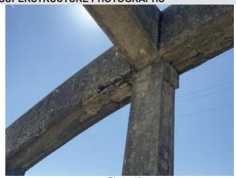
Photo 18 Spall in the left arch rib.
