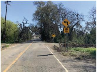
Photo 7 Vertical clearance 13 FT 6 IN and 15 MPH signs at the approach to Abutment 5.
