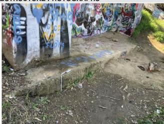
Photo 20 Exposed pile cap at Bent 2.
