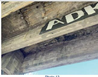
Photo 13 Vertical cracks in the girders in Span 1.
