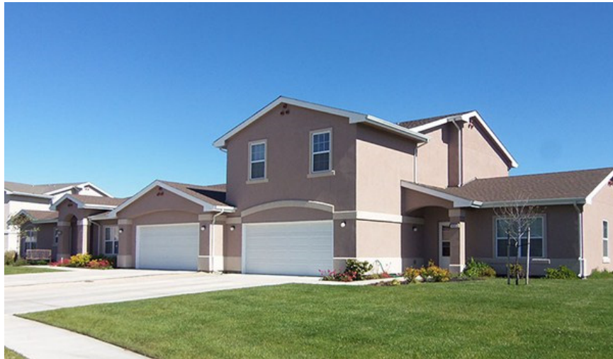
On-Base Housing at Travis AFB ( http://www.travisfamilyhomes.com/ )
