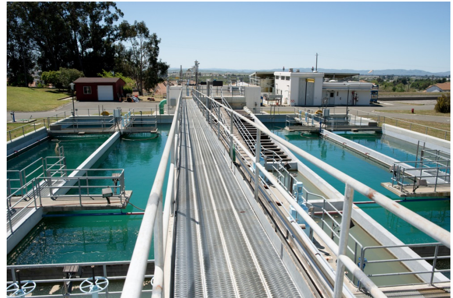
Travis AFB Water Treatment Plant
