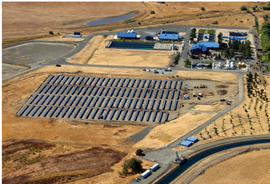
Solar array at North Bay Regional Water Treatment plant in Vacaville (Source: http://www.solarworld-usa.com/ )
