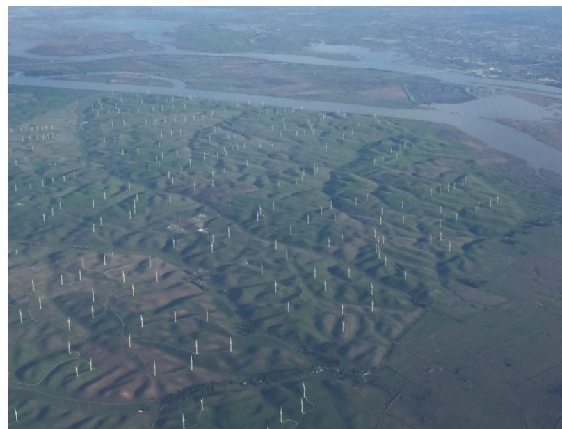
Montezuma Wind Energy Wind Farm
