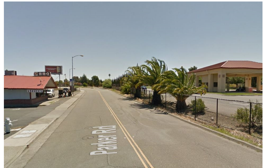
Minimal landscape screening and fence in front of the Main Gate along Parker Road (Source: Google Maps)
