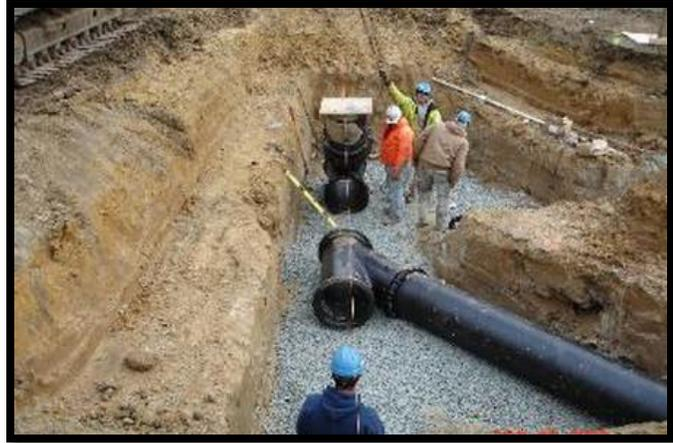
County Airport Road also in 2007. An 8-inch fire hydrant line and a 4-inch domestic line were also completed concurrently by the County. Extension and looping of water service lines will be necessary to further serve Airport development areas and will be evaluated within an updated Airport UMP.
