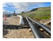
Last week, the temporary bypass line to provide water to Benicia began testing. This week, the first phase of testing has been successful and the structural integrity of the bypass line is sound. Testing will continue into next month when staff will try to expand the line to increase water flow.
