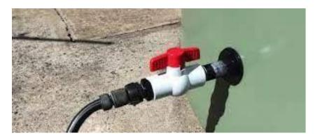
Watertight seal with attached ball valve on the side wall of a tank
