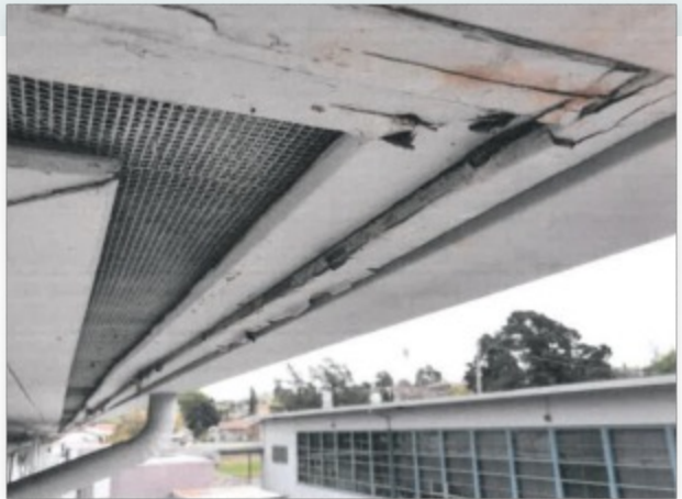
Signs of water damage can be observed at classroom roof soffits
