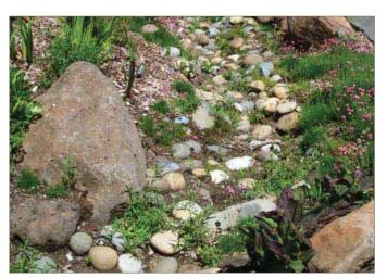
Figure 3-21: Vegetated swale increases infiltration and provides landscape feature
