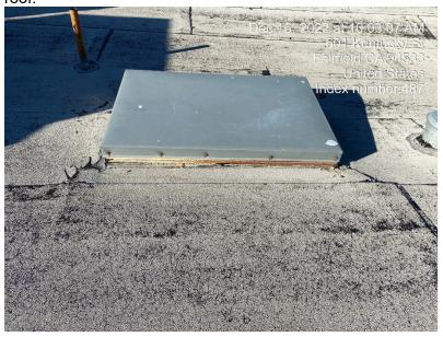
7. Replace existing galvanized sheet metal lid cover 2 each to match existing. Provide shop drawings to Solano County for approval. Show shop drawings how the lid will be remove and reinstalled similar to existing for County Approval prior to fabrication.
