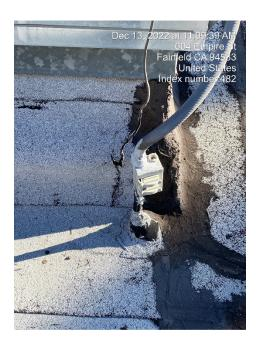
6. Keep existing galvanized sheet metal lid for future and extend sleepers 8 to 12 inches above existing roof.
