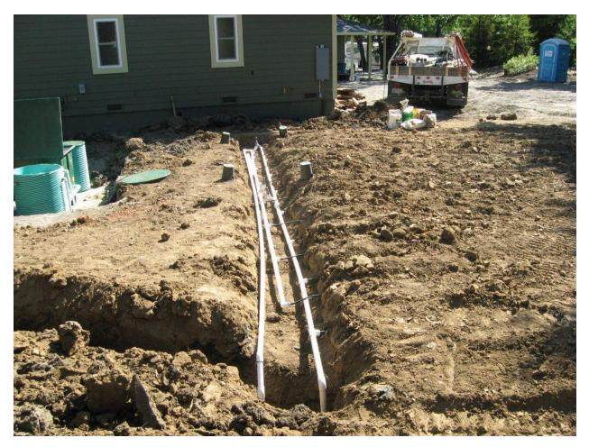
Example of the installation of a drip disposal field
